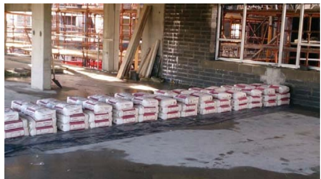
Figure 8. Load test on first floor slab
