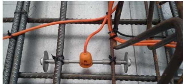
Figure 2. Vibrating wire gauge installed in the plate element.
