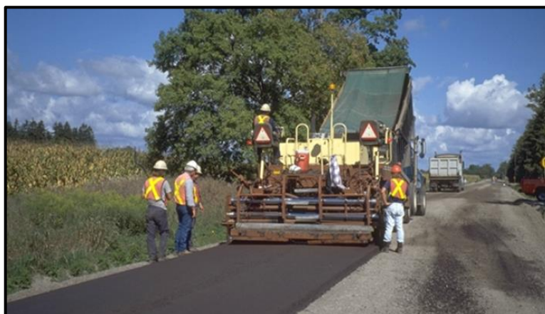
Figure 19: Laying (anionic) emulsion bound cold-mix in Canada [33]
