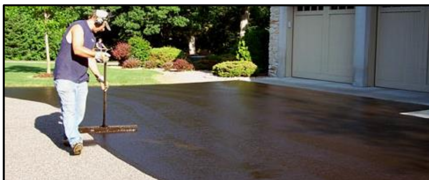
Figure 16: Driveway sealing by hand application [30]
