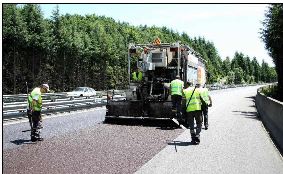
Figure 18: Applying a cationic micro-surfacing on a motorway in France
