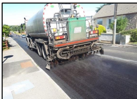
Figure 13: Tack coat application
