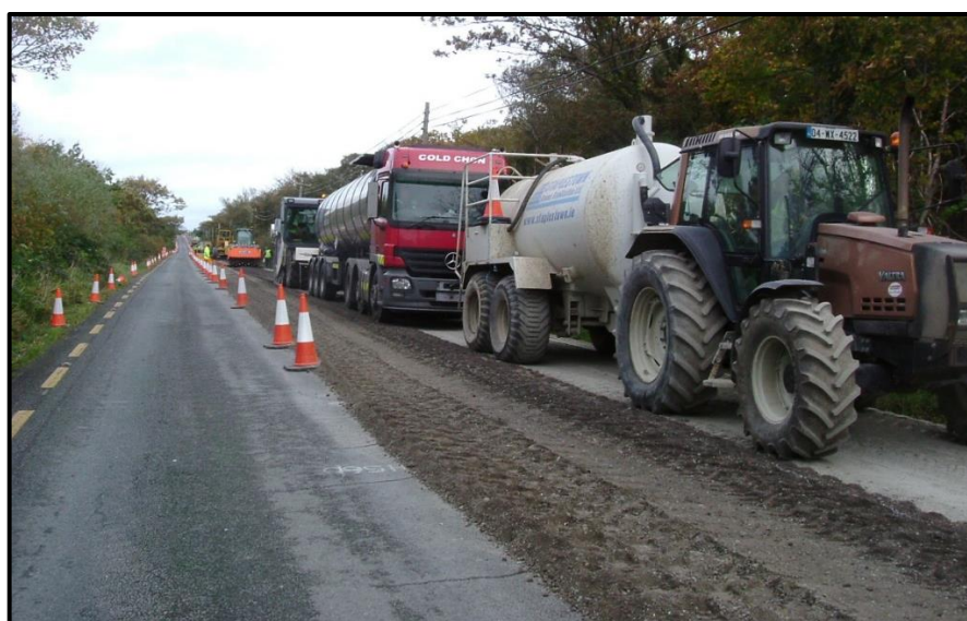
Figure 20: Sequence of machinery used for the cold in-place recycling process
