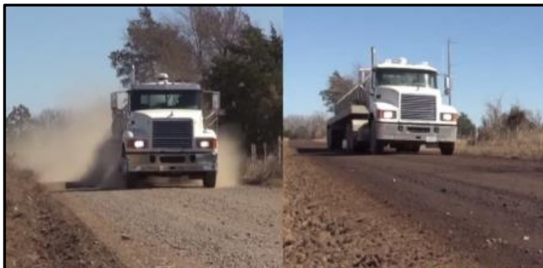
Figure 14: An untreated gravel road before and after a dust suppression emulsion is applied
