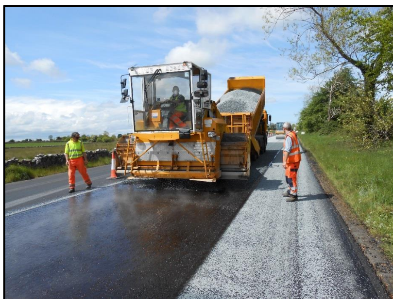
Figure 11: Applying the chipping to the surface dressing binder
